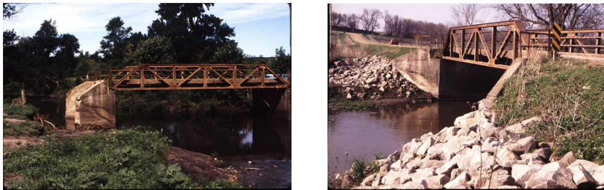
Figure 1.1 Effect of flood on erosion at a small bridge situated in Squaw Creek, close to Ames (Iowa). The left picture shows that all the erodible material behind the toe of the wing-wall abutment was washed by the flood. The right picture shows the bridge after the abutments were reconstructed and riprap stone was placed on the floodplain around the abutments
